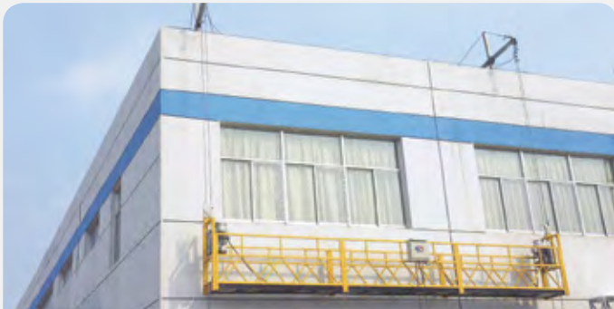
Temporarily installed Suspended Access Equipment - Platform
