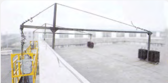
Temporarily installed Suspended Access Equipment - Suspension Mechanism
